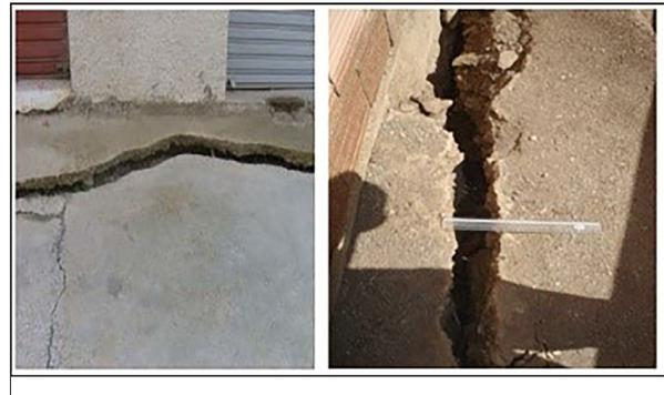
Figure 19. Failure mechanism 2 (finite difference analysis with a high piezometric height).
